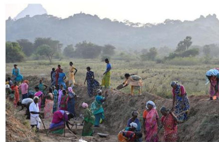
Right to work: People employed under the MGNREGA scheme dig a trench in Tiruvannamalai, Tamil Nadu. C. VENKATACHALAPATHY
