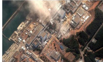
The No. 3 nuclear reactor of the Fukushima Daiichi nuclear power plant burning after the earthquake and tsunami triggered an explosion. Satellite image taken March 14, 2011. DIGITALGLOBE
