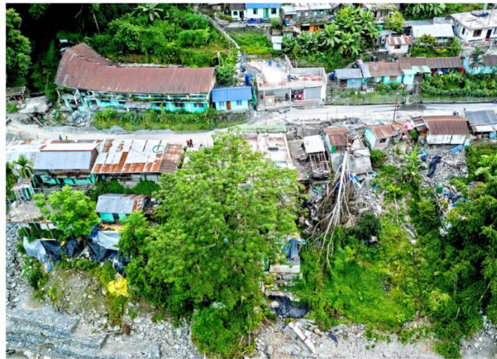
A view of Teesta Bazaar in West Bengal, which has been sinking further into the ground since the glacial lake outburst flood in 2023. SPECIAL ARRANGEMENT
