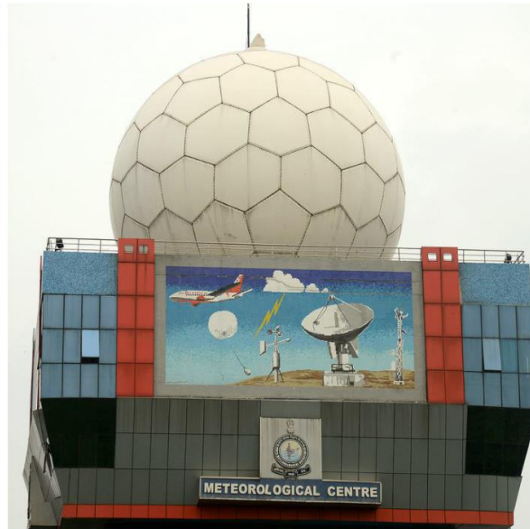
Weather blues: The complex housing an S-Band Doppler Weather Radar at the Meteorological Centre in Begumpet, Hyderabad. FILE PHOTO
